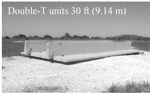
Figure 5. Double-T sill dimensions and placement configuration
