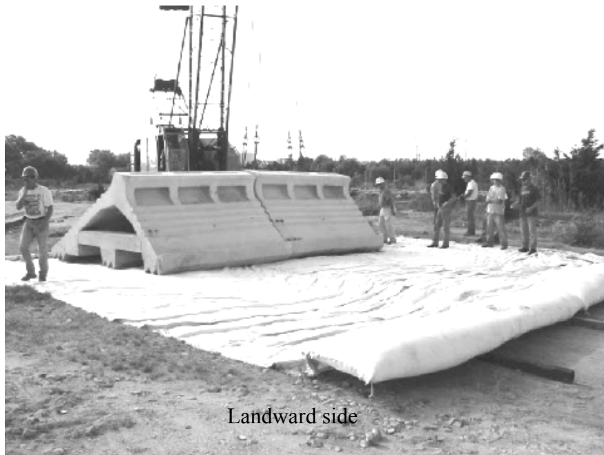
Figure 4. Geotextile fabric mat base for Beachsaver Reef™
