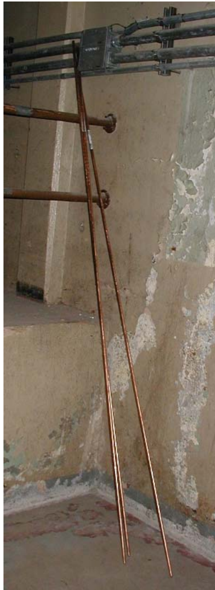
Figure 22. Copper clad grounding rods.
