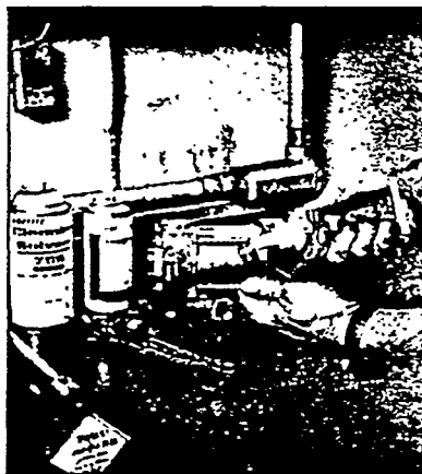
Sealant is applied to pipe threads of air inlet to actuator cylinder.
