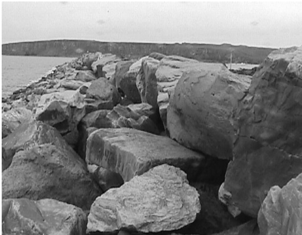
Figure 1. View of St. Paul Harbor breakwater trunk
