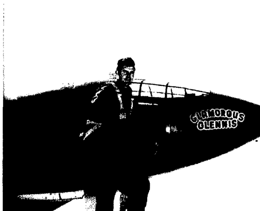
Charles E. Yeager in the late 1940s. He is wearing a standard flight suit, seat parachute, and holding a hard shell helmet. The flight suit was made of cotton and would burn. The later nylon flight suits were quickly removed from service, as they would melt and stick to the pilot's skin, causing severe burns. The hatch in the side of the X-1 was useless for an in flight escape, as it was forward of the wing. Air Force photo
