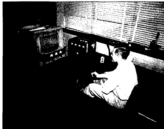
The X-1B simulator in 1958. The display is a cathode ray tube, while the cockpit is a large wooden box. NASA photo
