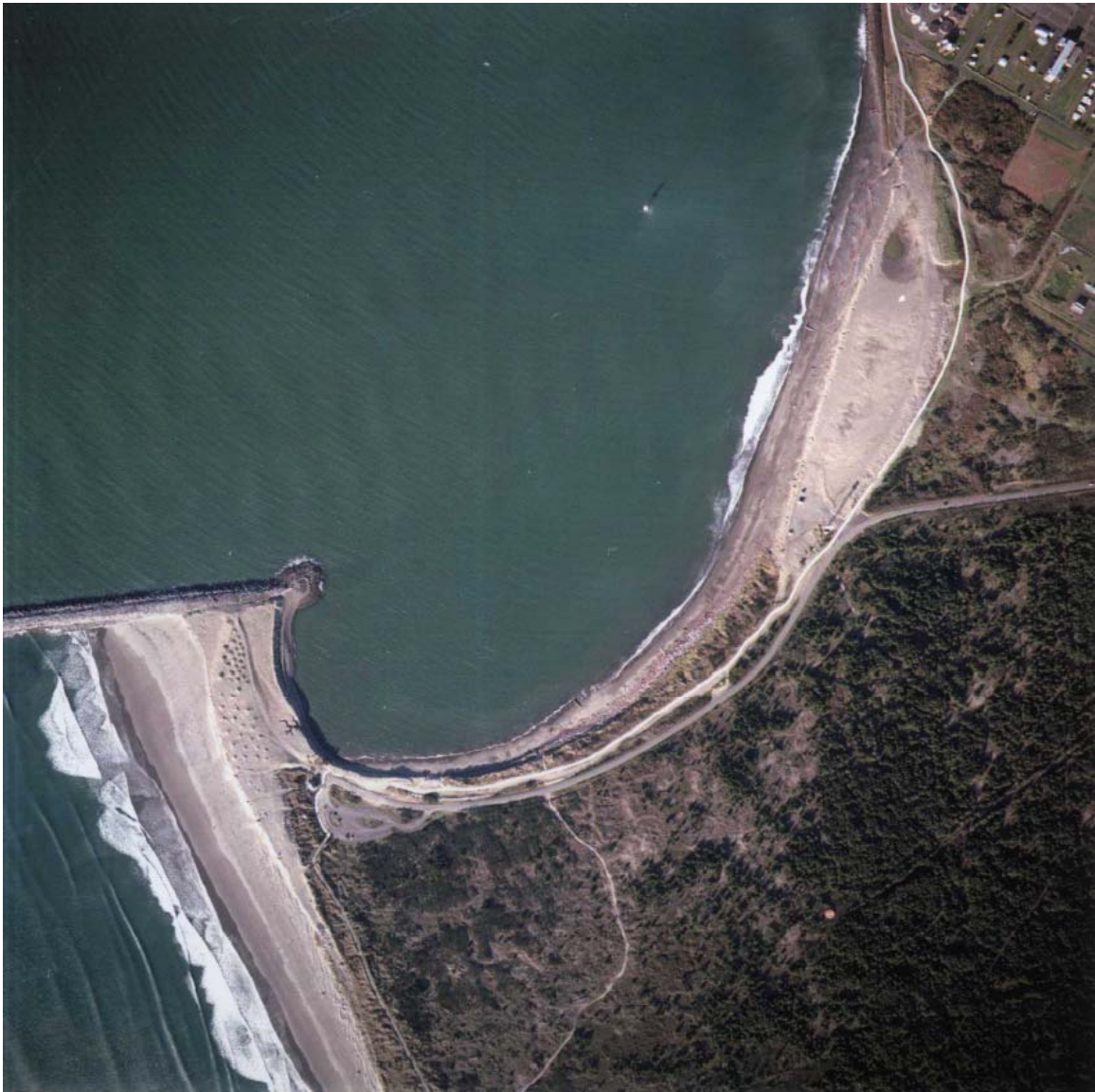
Figure 3. South jetty and shoreline of Half Moon Bay, 31 October 2003.
