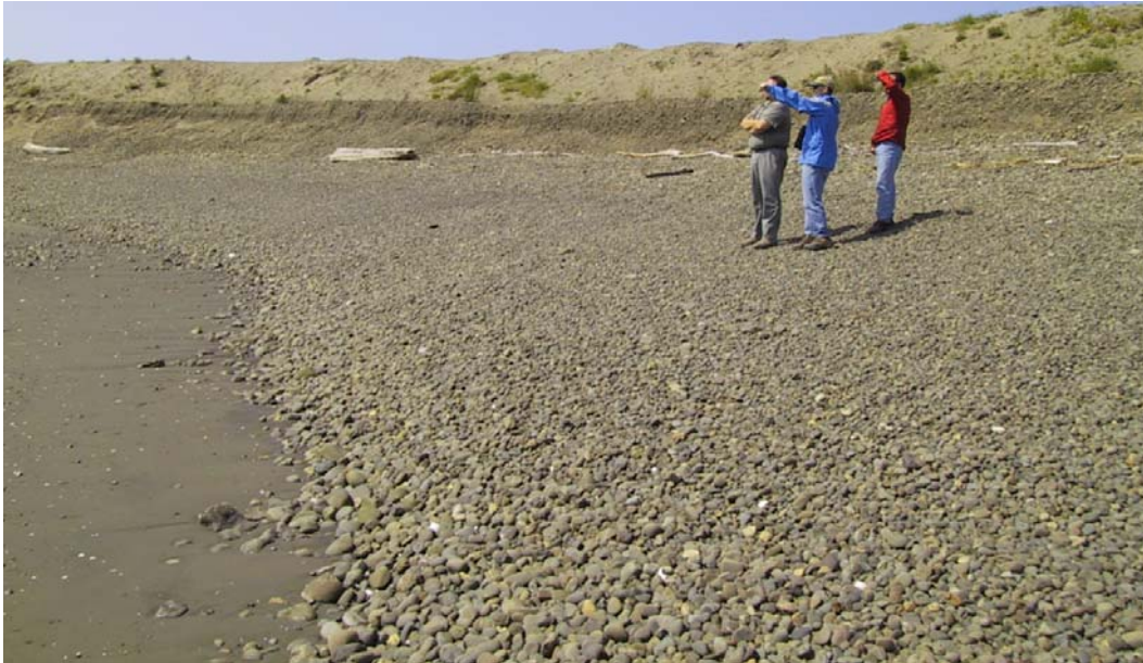
Figure 5. View of transition gravel protection from diffraction mound.
