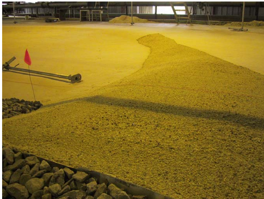
Figure 22. Placed gravel transition looking southeast from south jetty.
