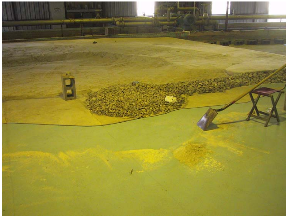
Figure 15. Construction of diffraction mound at eastward end of south jetty.
