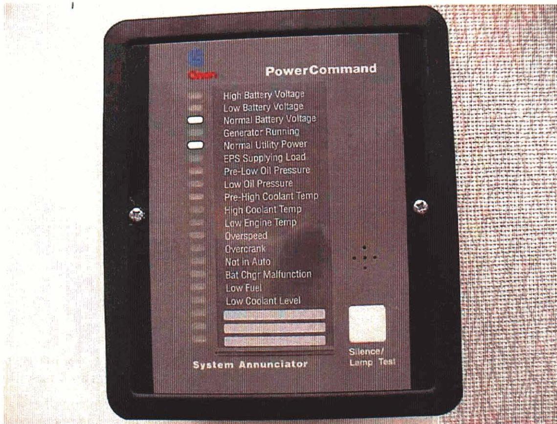
Figure 16. Remote Instrument Panel for Emergency Generator
