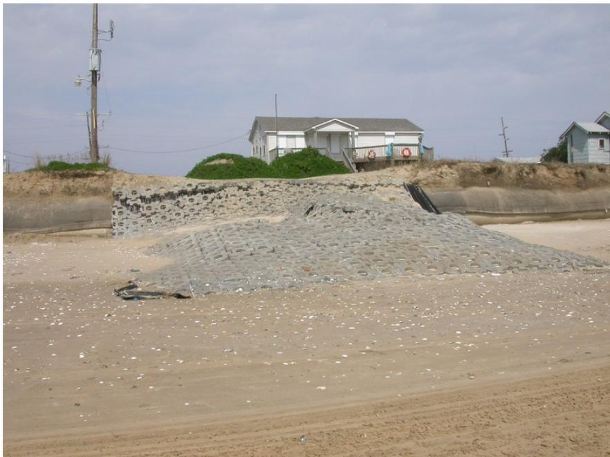
Figure 27. Dune protection north of Rollover Pass (19 February 2003). These interlocking concrete units have been placed over sand-filled fabric tube.
