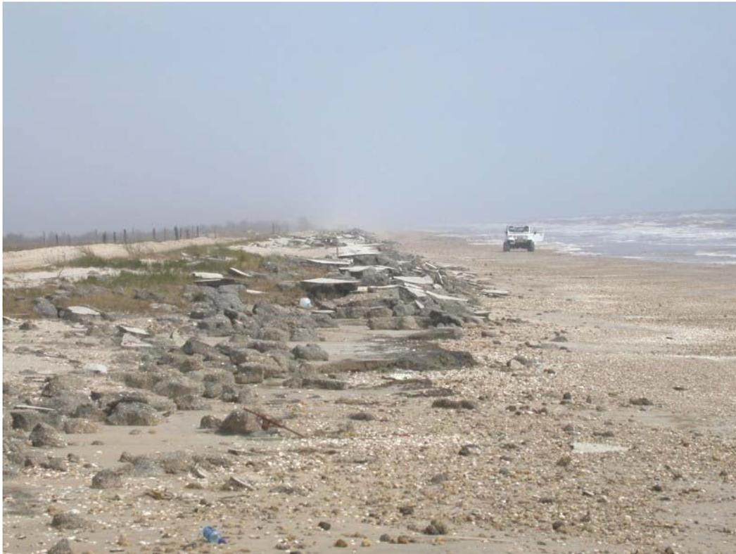
Figure 24. Broken pavements, remnants of State Highway 87, near west end of McFaddin NWR. Day this image was taken, beach was completely covered with sand, shell hash, and gravel (19 February 2003).
