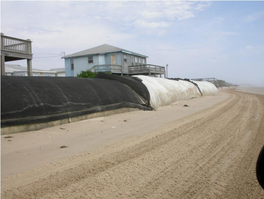
Figure 28. Sand-filled fabric tubes protecting dunes and homes west of Rollover Pass (19 February 2003).
