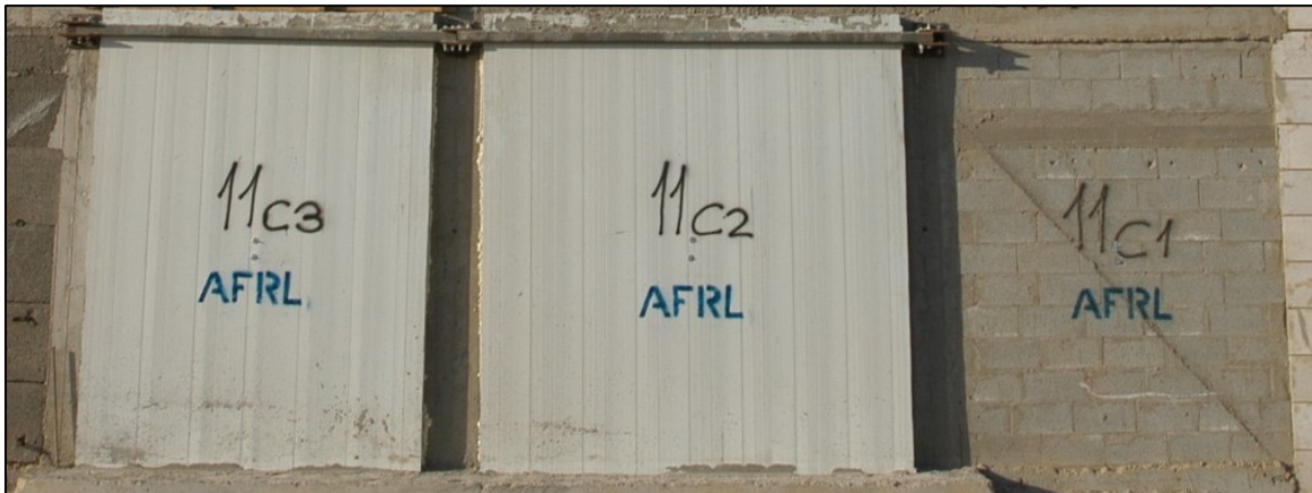
Figure 16: Experiment 2 Pre-Detonation (4", 6" & 4" Behind CMU)
