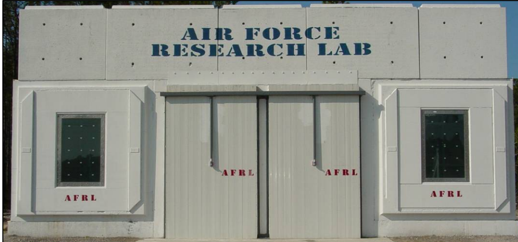
Figure 15: Experiment 1 Pre-Detonation (8" & 8" Insulated)
