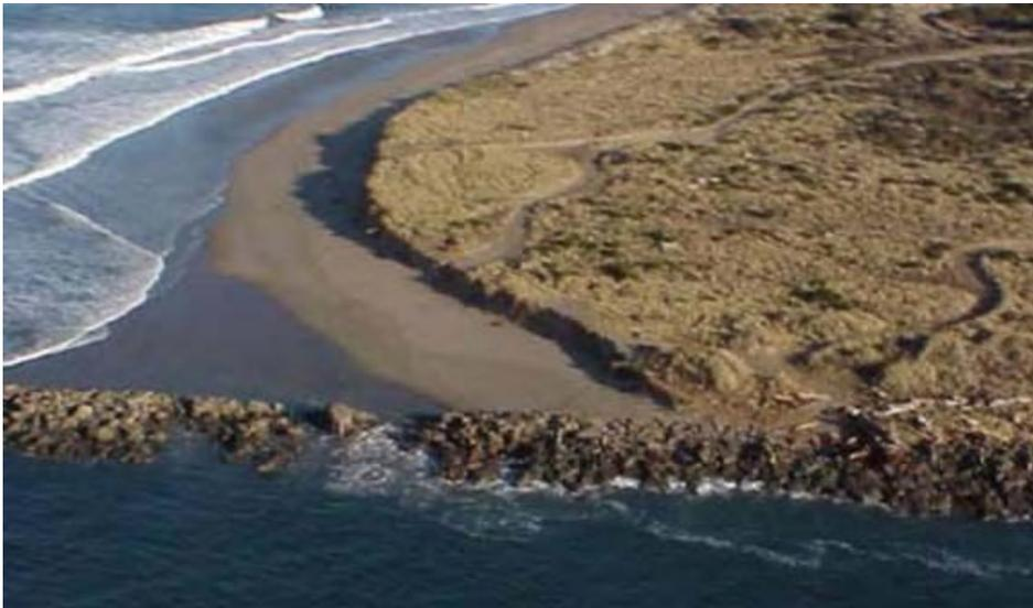
Figure 100. Degraded north jetty at Coos Bay, OR, and inception of flanking channel expected to lead to a breach (December 2002; photograph by U.S. Coast Guard)
