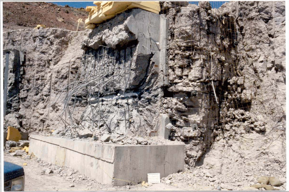
Figure 14. Test 3, Shot 1, resulting damage to Panel 3.
