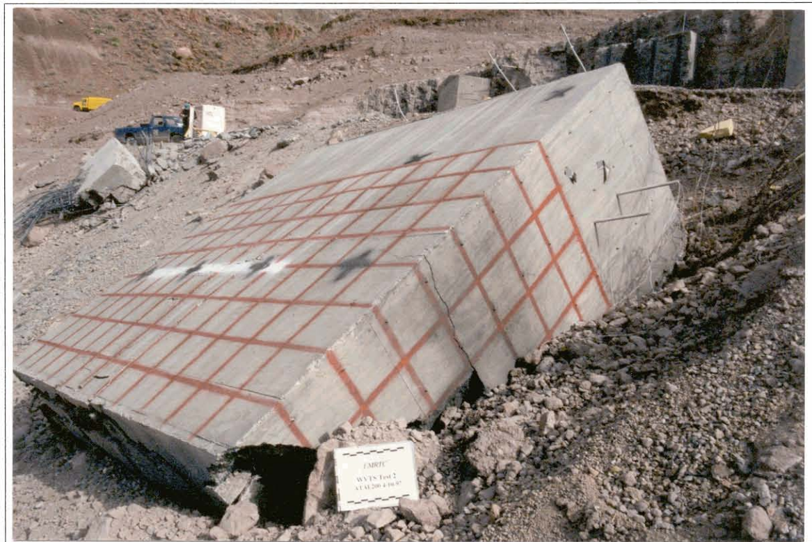
Figure 9. Resulting damage to Panel 2.
