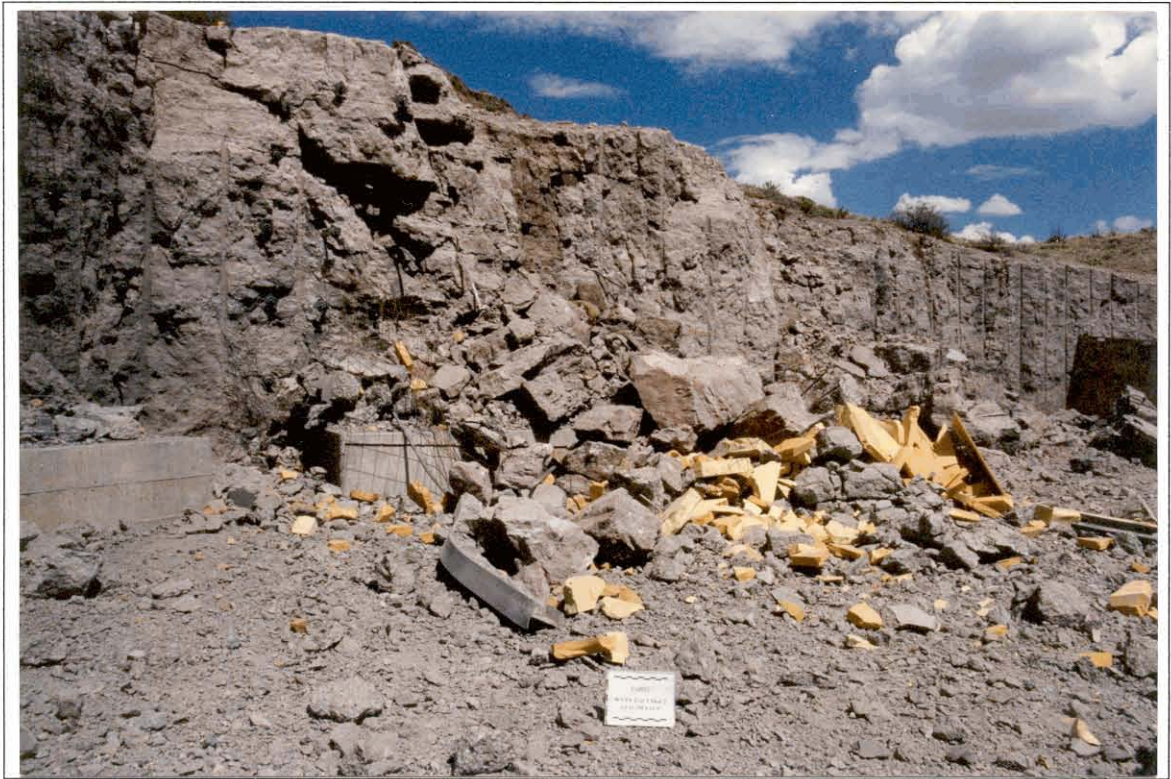
Figure 15. Test 3, Shot 2, resulting damage to Panel 3.
