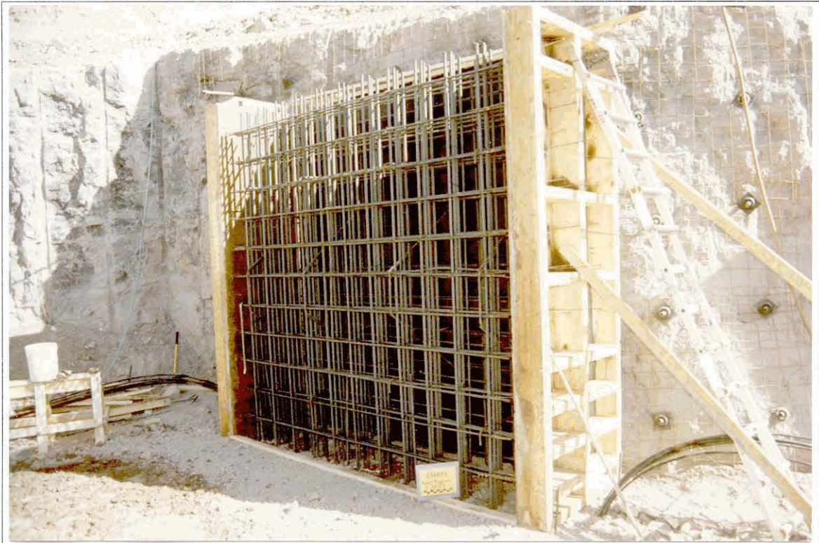
Figure 2. Reinforcement bar placement prior to concrete placement.
