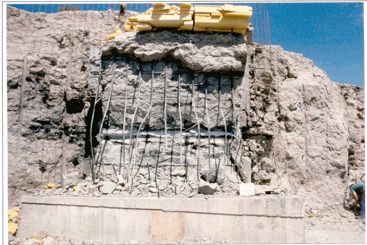
Figure 13. Test 3, Shot 1, resulting damage to Panel 3.
