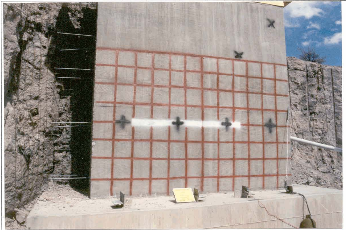
Figure 8. Panel 2 charge placement (indicated by white bar on panel face).
