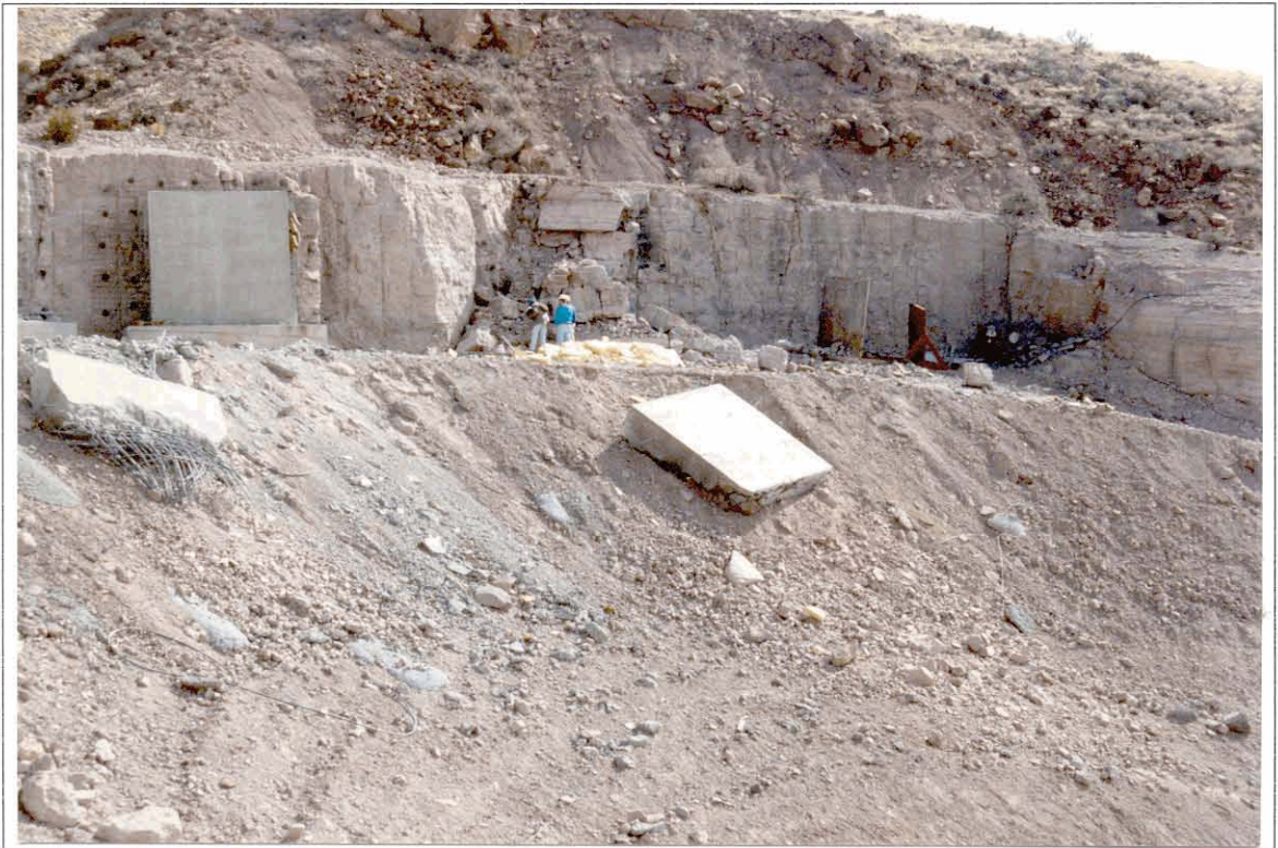
Figure 10. Resulting damage to Panel 2.
