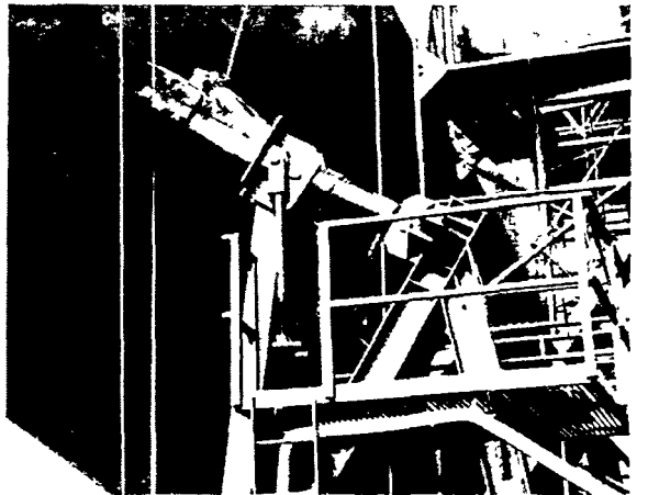
Fig. 13c. Hydraulic Jig for Joining of Sub-blocks
