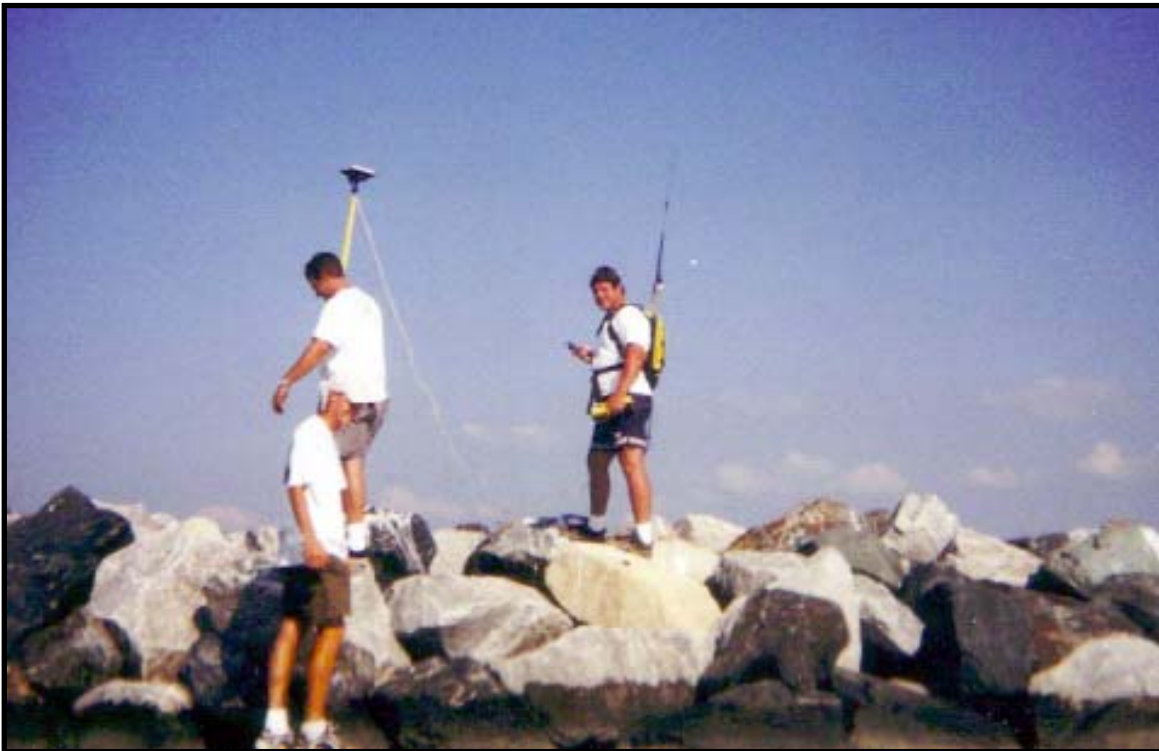
Figure 23. Breakwater survey team using RTK-GPS equipment, with construction adhesive and paint as stone marker points for repetitive surveying (after Pratt 2003).
