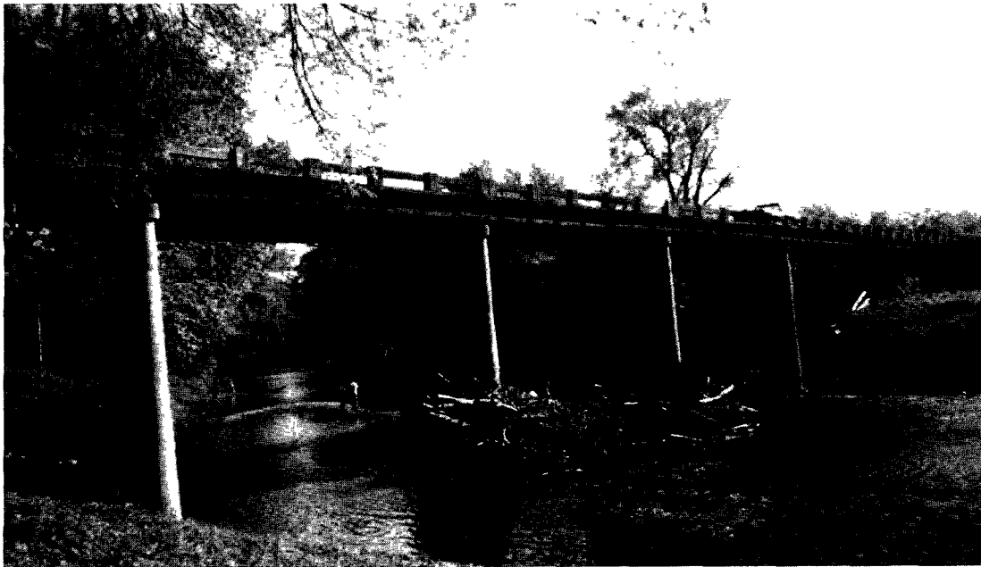
Debris accumulation at bridge over the Harpeth River at Sneed Road near Bellvue, Tennessee.
