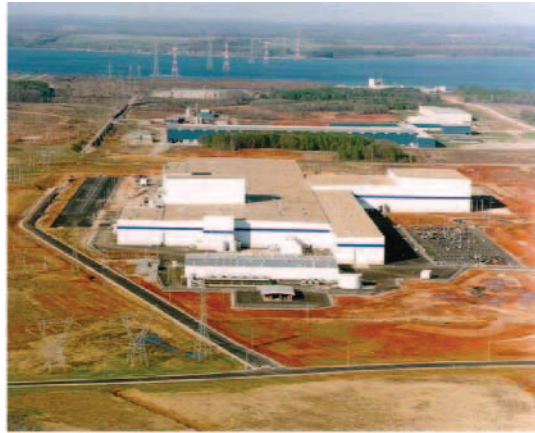
Figure 3.6 Delta IV Assembly Facility in Decatur, Alabama
