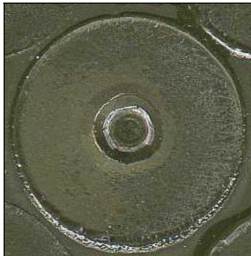
Figure 10. Typical cohesive failure of the topcoat applied over MIL-P-53022 primer.
