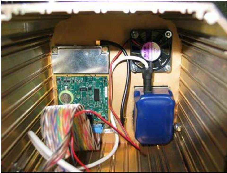
Figure 3.2: Inside Back-plate of Test Unit
