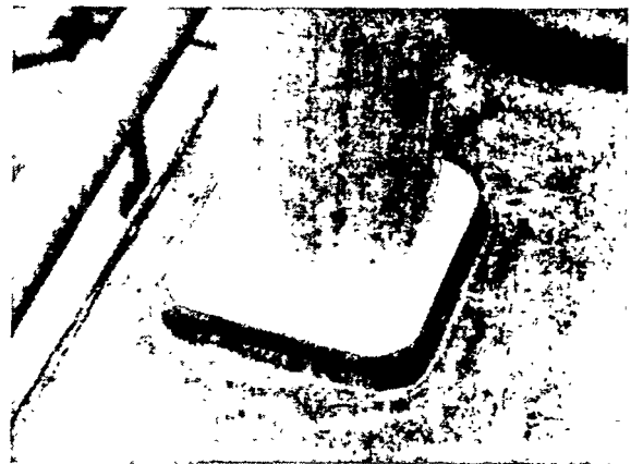
FIGURE 6: Stanchion support transition joint steel fillet weld is made to vertical edge of pad.
