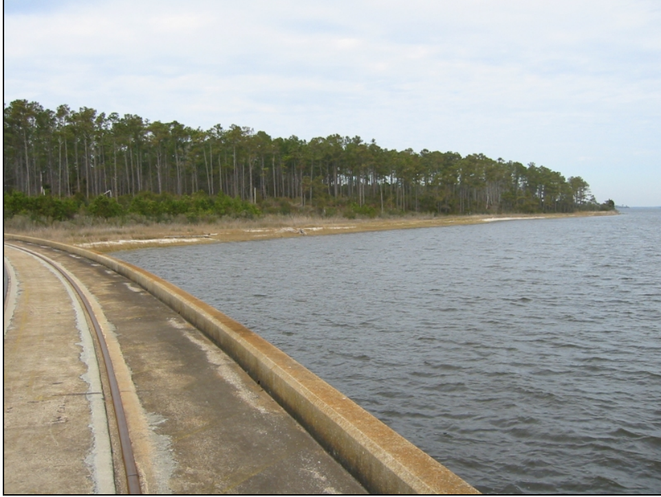
Figure 15. Sunny Point Terminal south wharf, view looking north. A boat ramp is located at point of land in right side of photograph dated 1 February 2005
