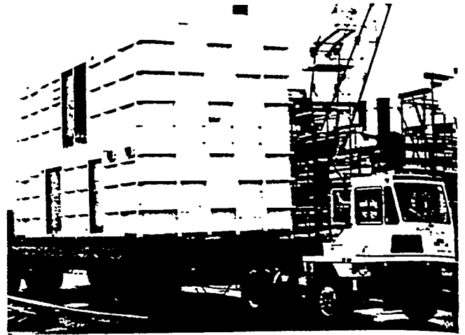
Fig. 3 Grand block being transported to ship. (Does it matter where the ship is??? Can we look forward to government-furnished manufacturing?)
