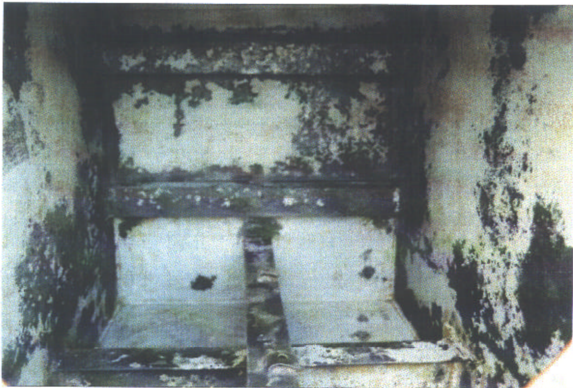
PHOTOGRAPH 4-POWER/HAND TOOL CLEANED SURFACE PRIOR TO COATING
