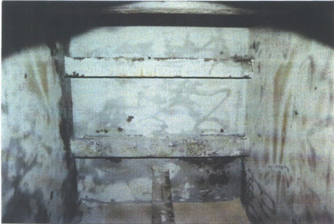
PHOTOGRAPH 3-SWEEP BLAST CLEANED SURFACE PRIOR TO COATING
