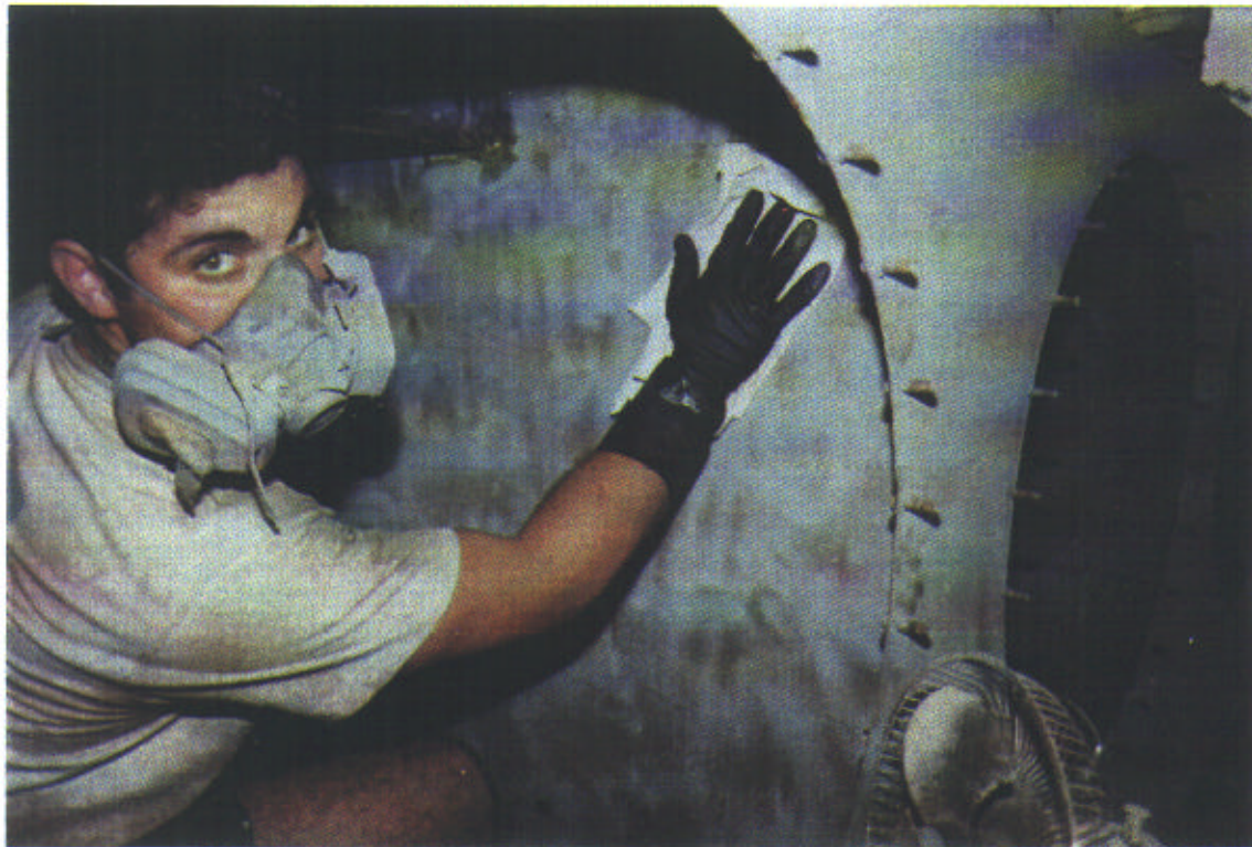
PHOTOGRAPH 5-SURFACE PREPARATION OF INTACT MIL-P-24441
