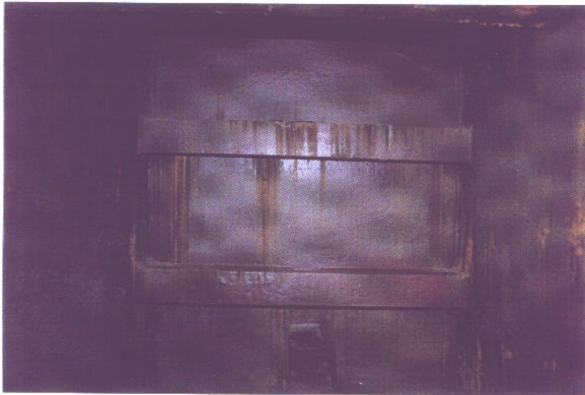
PHOTOGRAPH 10-REPAIRED SURFACE TOLERANT EPOXY "B"
