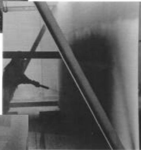
Figure 1-7: Blast cleaning in a confined space using coal slag abrasive; note high dust level and poor visibility.
