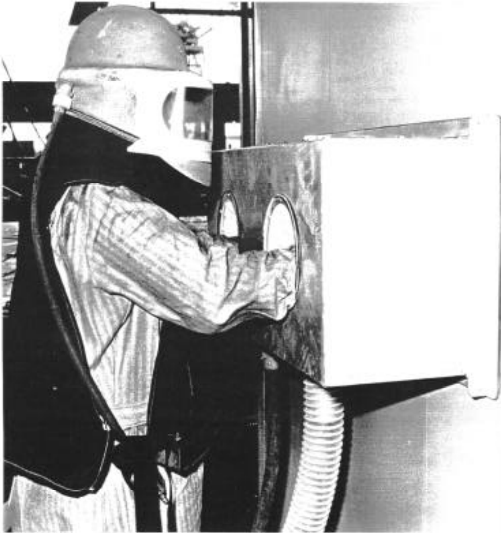
Figure 2-11 Small Area Blaster in use on a vertical surface. Note lack of dust and abrasive escaping from containment.
