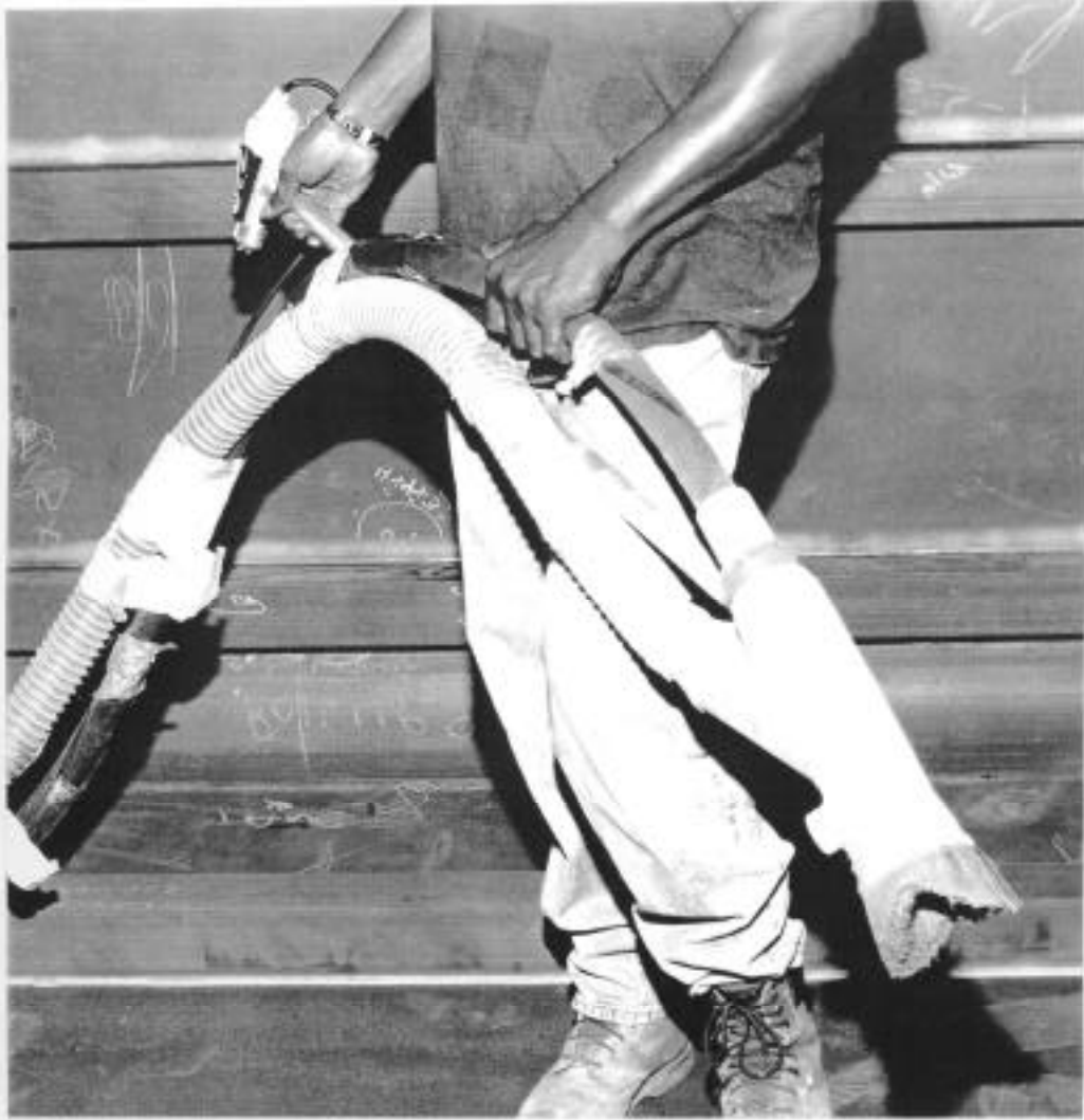
Figure 2-1 The vacuum-blast head assembly and weld areas blast cleaned with the vacuum-blast unit.
