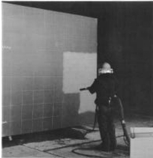
Figure 1-6: Blast cleaning in a confined space using steel abrasive; note lack of dust and good visibility.
