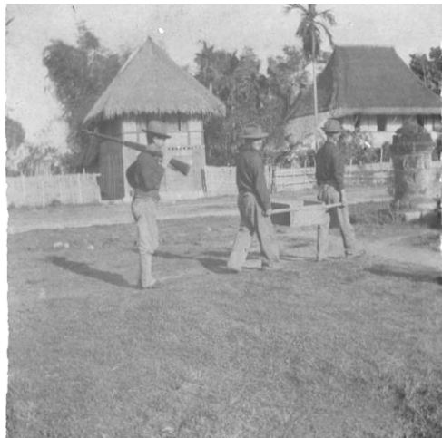
Figure 16. Privates Killingsworth, Bridges and Jordan (G Company) working on a construction project. Source: Archives of the 32nd Infantry Regimental Association.
