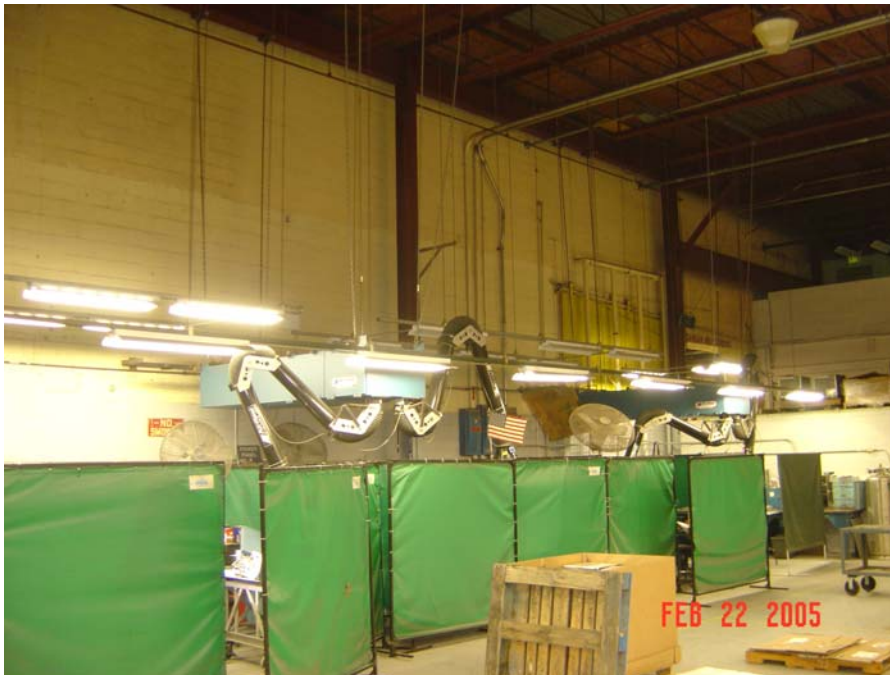
Figure 12. Building 1A welding area.
