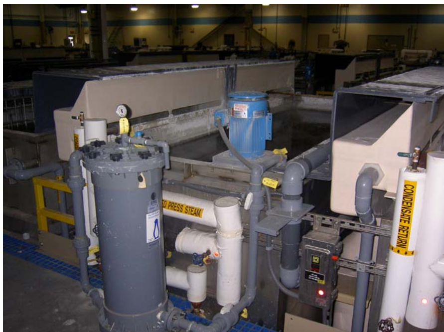
Figure 6. Plating tank push-pull exhaust system.
