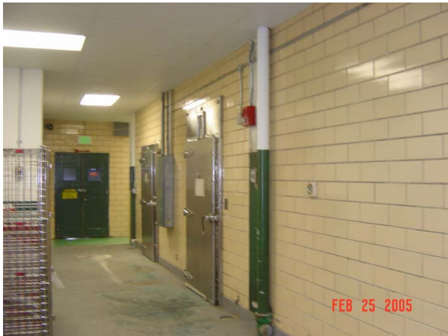
Figure 28. Walk-in cold storage freezer units.
