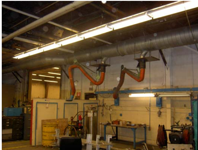
Figure 14. Welding exhaust in Building 14.
