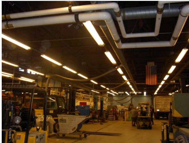
Figure 16. Exhaust from vehicles in motor pool, Building 15.
