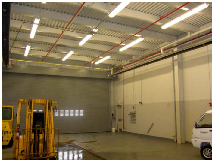
Figure 20. Building 15 vehicle washing room.
