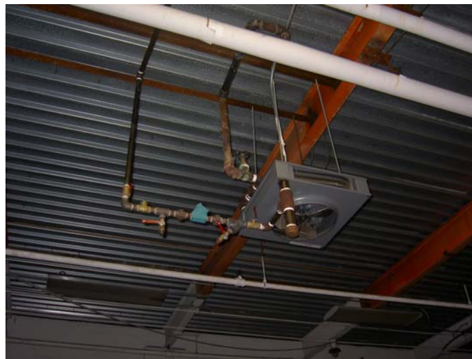
Figure 23. Heater in Building 1C Bay 6.
