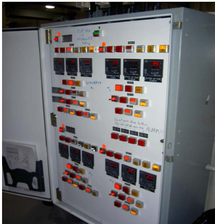
Figure 4. Plating Shop ventilation control panel.
