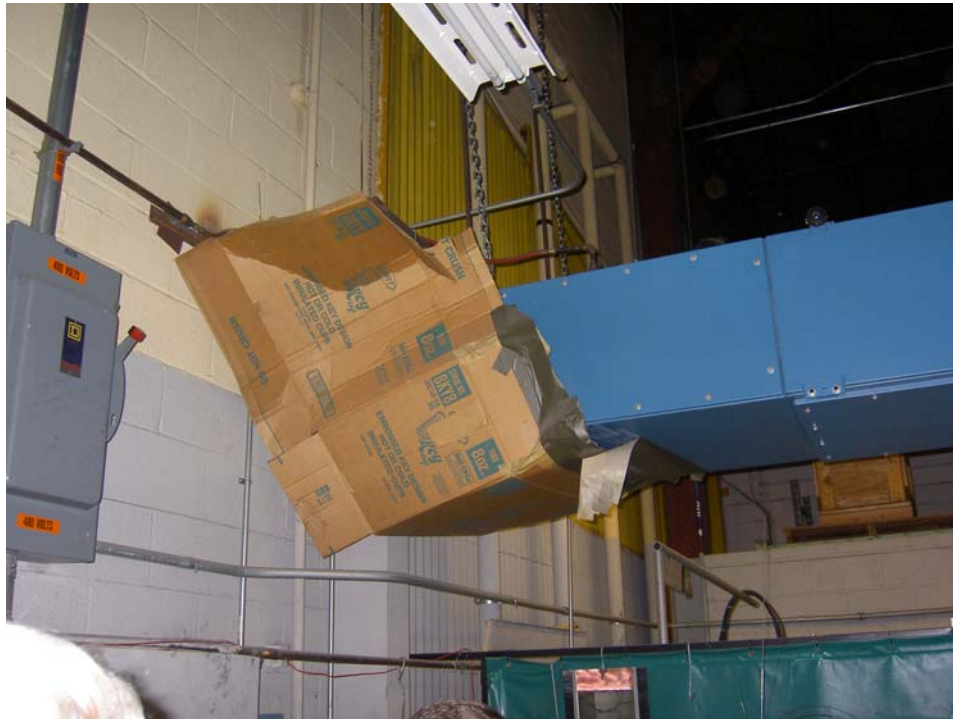
Figure 13. Carton used in B-1A Welding Shop to protect from air flow and noise
