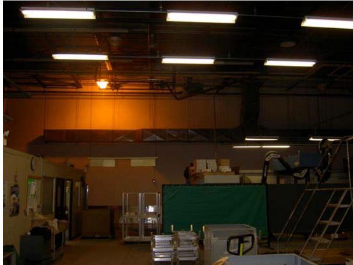
Figure 17. Welding supply air system in Building 1A.
