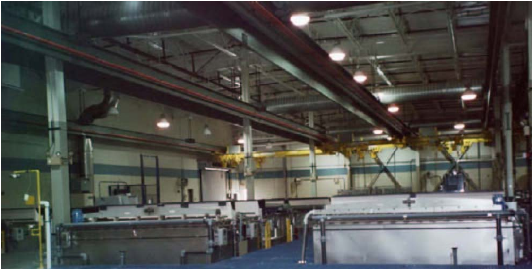
Figure 2. Plating Shop in IOF.
