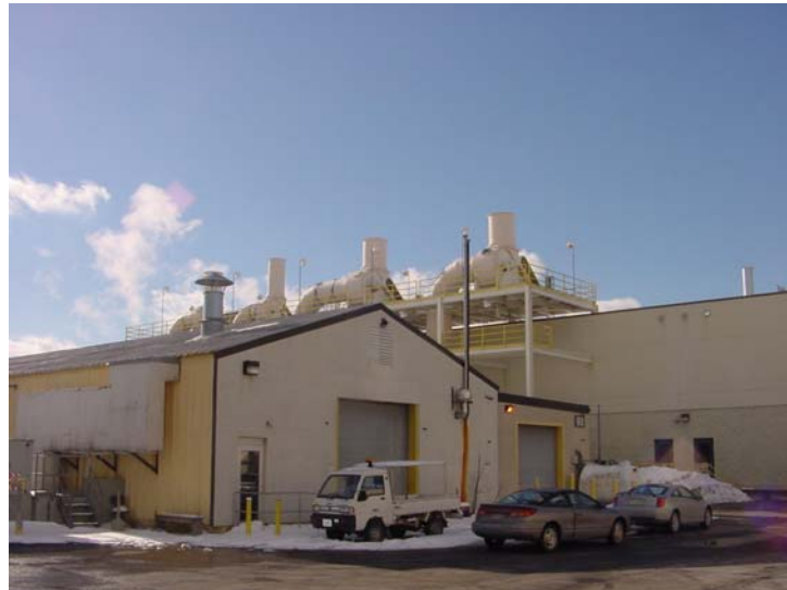
Figure 9. Steam plume from IOF roof-top.
