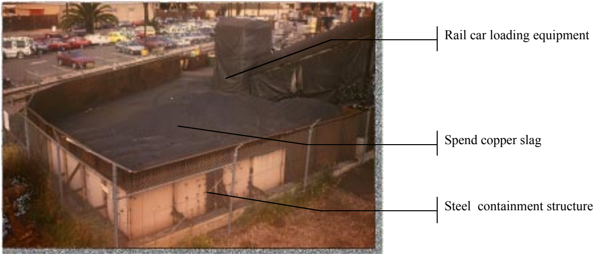
Figure 4: Spent Abrasive Storage - Copper Slag
