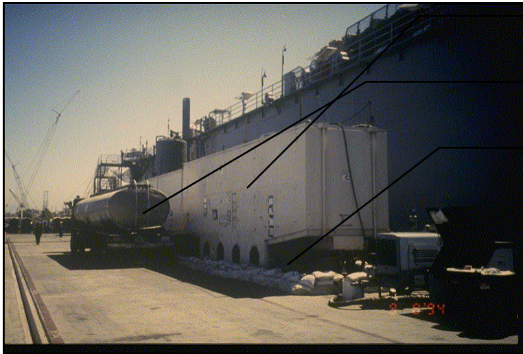
Figure 10: Oil/Separation tank - gravity Separation
