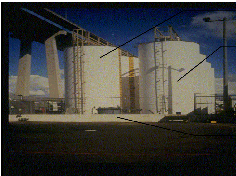
Figure 12: Oily/water storage tanks and treatment facility
