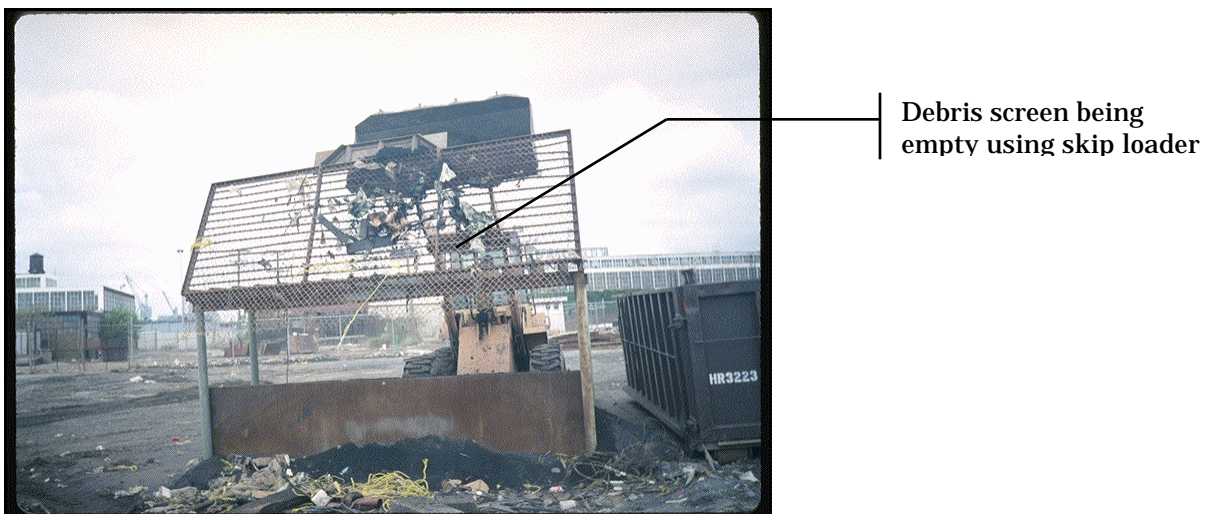
Figure 3: Removal of debris after screening
