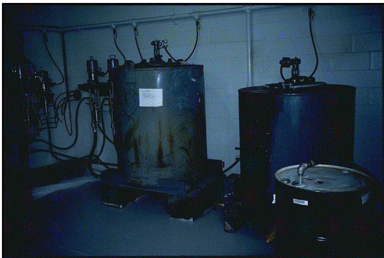
Figure 14: Stationary plural component paint mixing system
