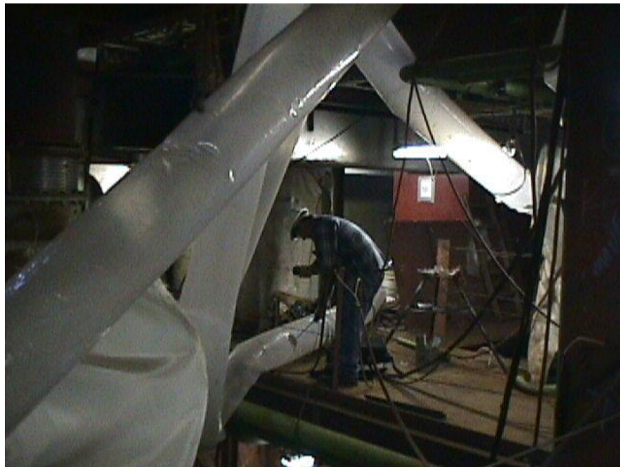
Photograph 1. Pneumatic powered portable ventilation fan propped over tank hatch cover aboard ship under construction
