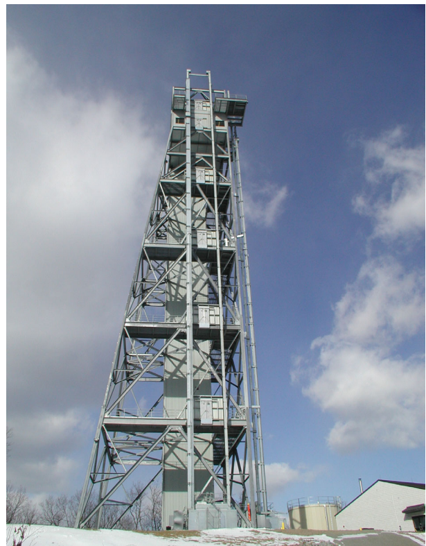
Fig. 1. PAL measurements tower.
