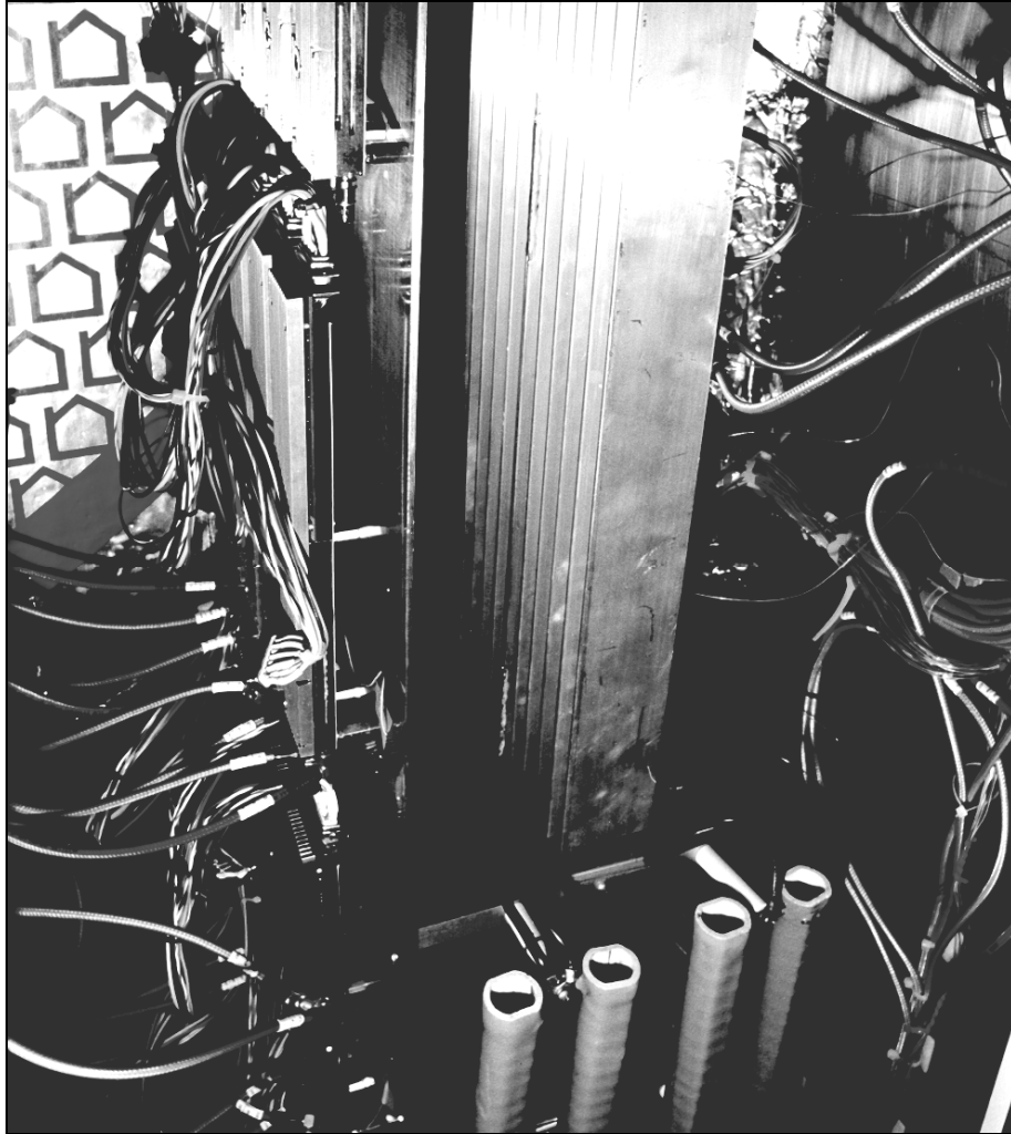
FIGURE 3.2.4 – C BAND T/R MODULES IN LIFE TEST CHAMBER (LEFT SIDE)
