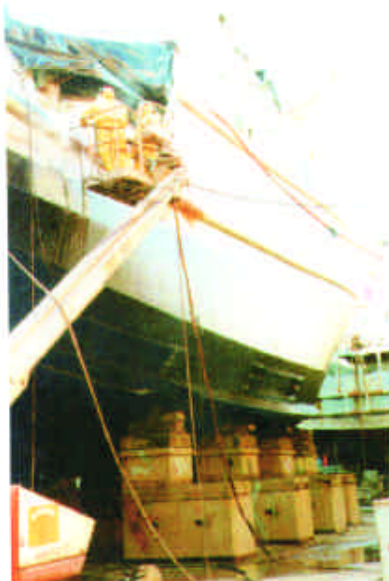
Figure 8: Operator and helper using UHPWJ
