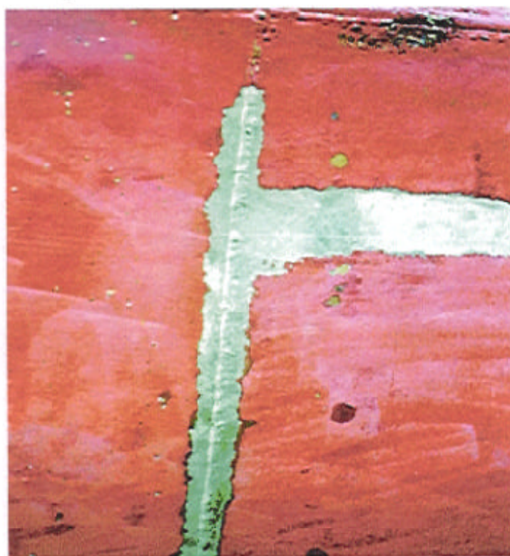
Figure 12: Spot removal by needle gun prior to complete section removal and replacement.
