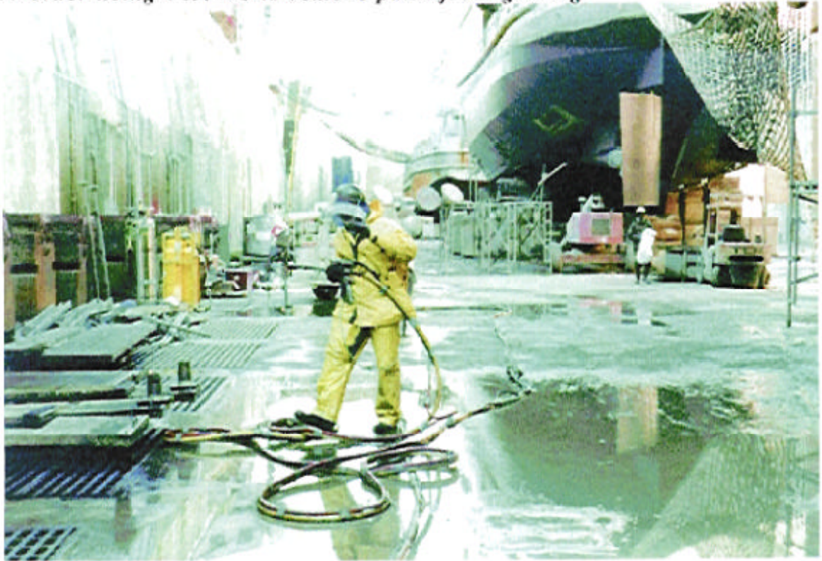
Figure 11: Worker using UHPWJ to remove paint from grating.
