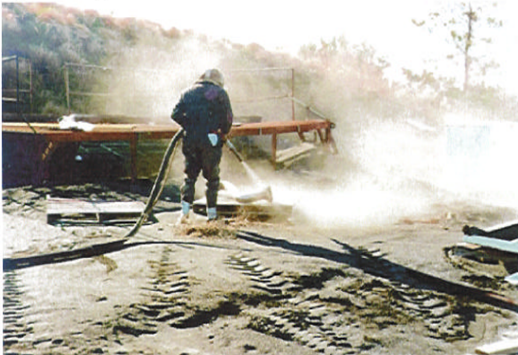
Figure 17: Type CE Abrasive Blast Helmet in use during OAAB.
