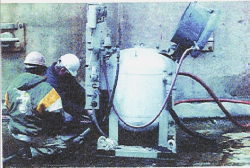
Figure 24: Workers adjusting Low Volume Slurry Blasting (LVSB) unit.
