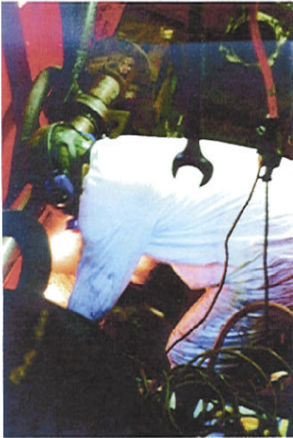
Figure 14: Needle gun in use cleaning primer coating and welding slag.
