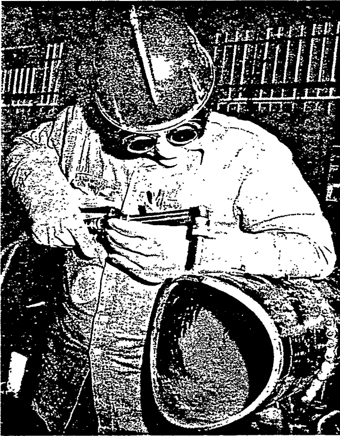
Manual contour burning process.
