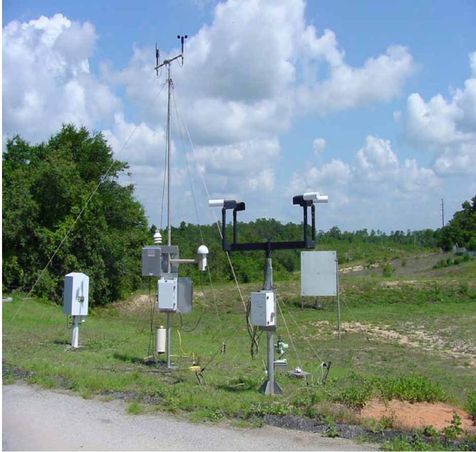
Figure 12. Picture of the RAWS at site C-72.
