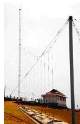
Fig. 2. A view of one transmitting antenna.
