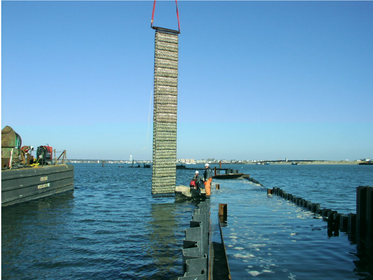
Figure 12. Mattress placement at Seabrook, NH, Section 227 project (photograph by Scott Leonard, New England District)
