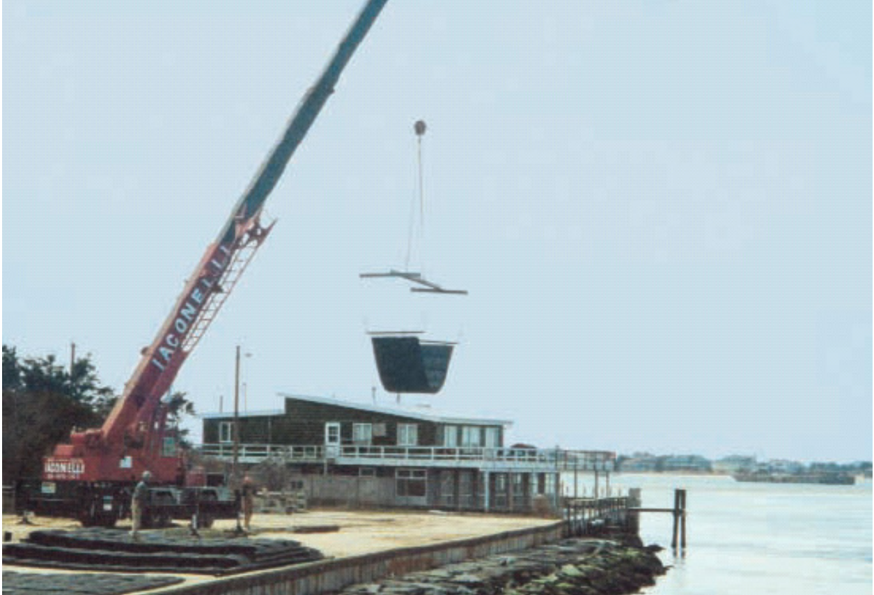
Figure 3. Installation of mattress at Barnegat Inlet, NJ (photograph courtesy of Tensar Earth Technologies)
