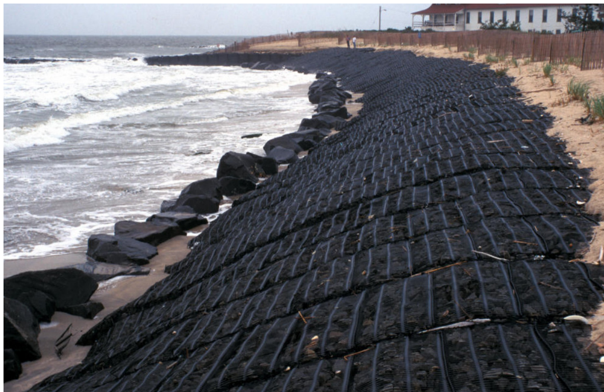
Figure 7. Cape May State Park shore protection mattress revetment shortly after placement (photograph from Jeffrey Gebert, Philadelphia District)
