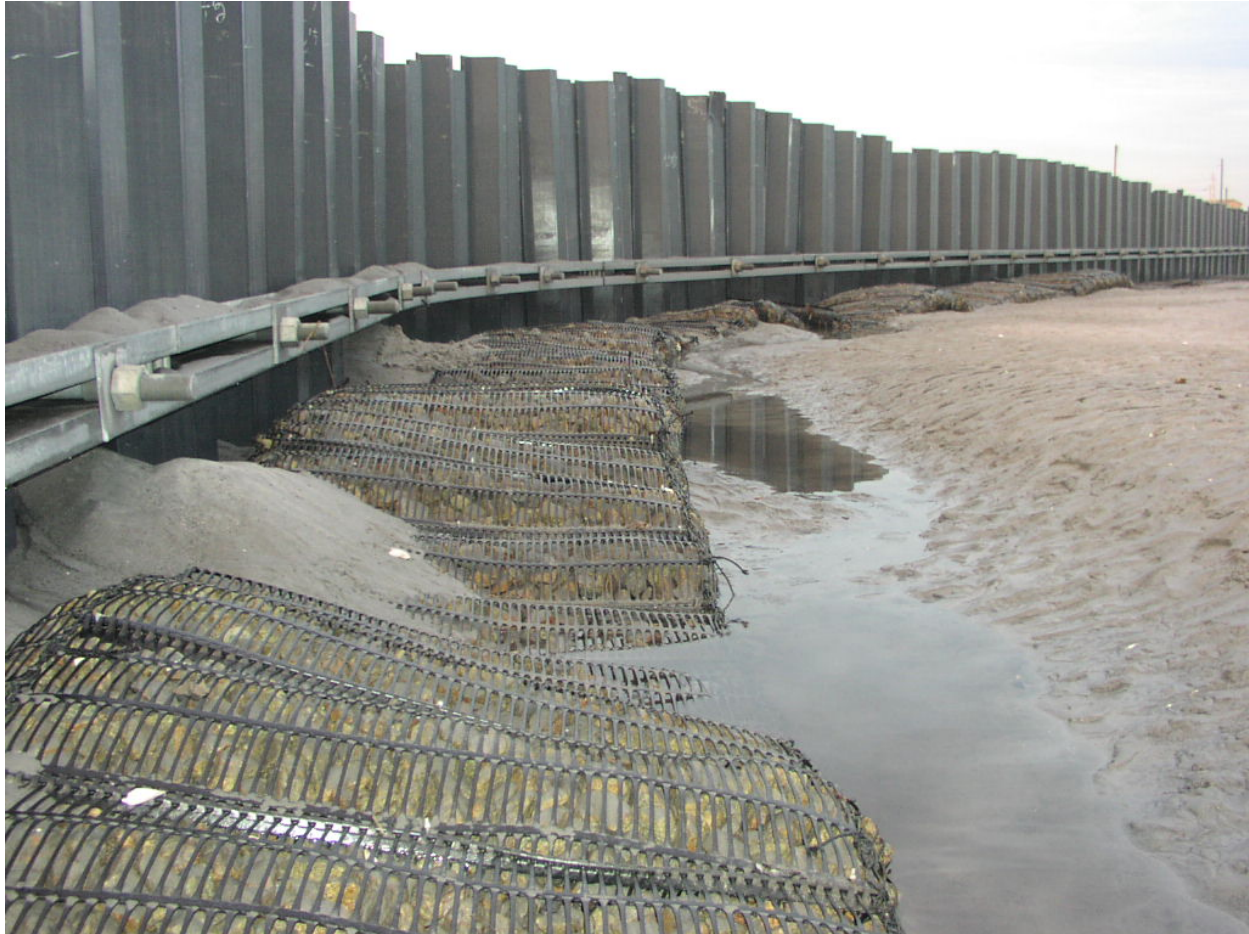
Figure 13. Scour apron at Seabrook Section 227 project at low tide (photograph by Scott Leonard, New England District)
