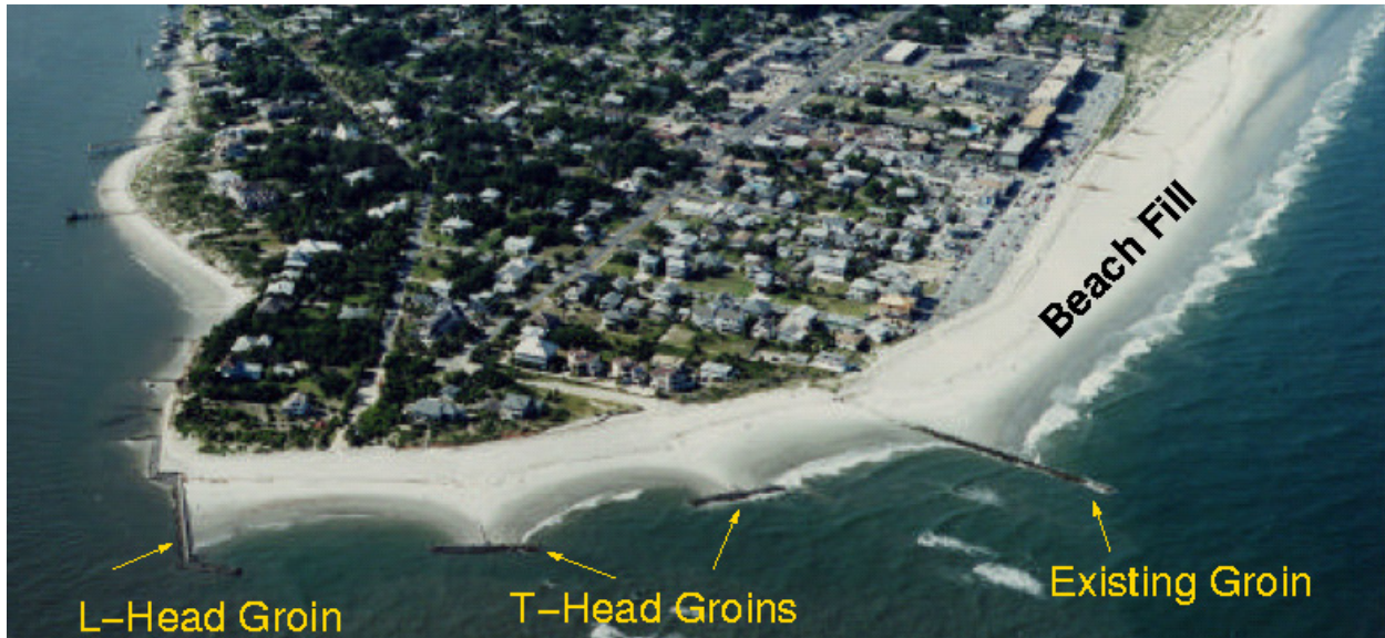
Figure 10. Terminal groin field at Tybee Island, GA (photograph courtesy of Olsen and Associates, Inc.)
