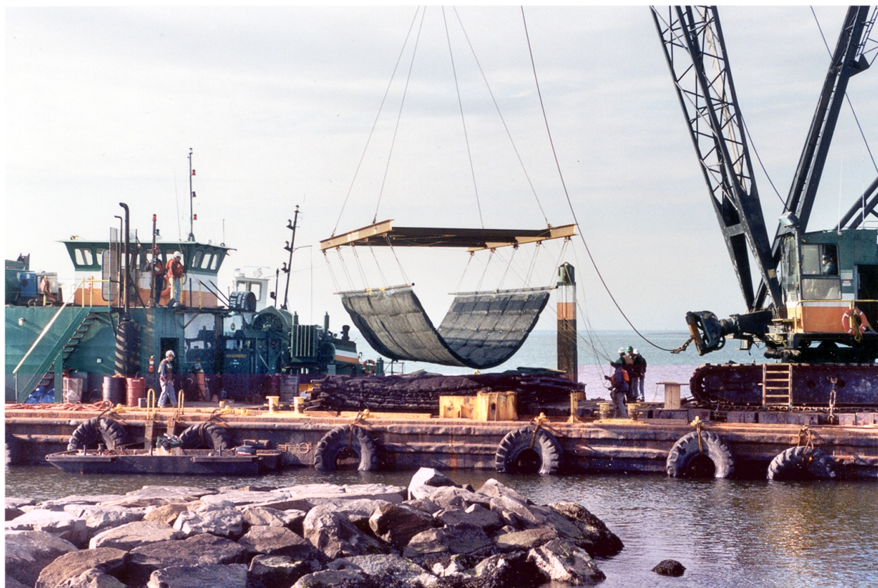
Figure 9. Barnegat Lighthouse with mattress placement underway (photograph provided by Jeffrey Gebert, Philadelphia District)
