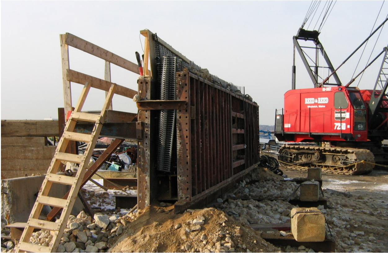
Figure 6. Construction jig used to fill marine mattresses at Section 227 project in Seabrook, NH (photograph by Kevin Knuuti, CHL)
