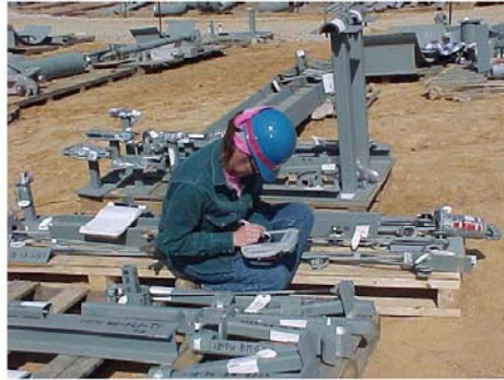
Figure 1: Worker Receiving Pipe Support using RFID Approach
