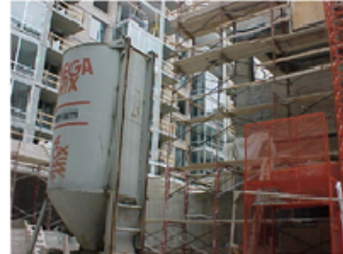
Typical site condition for inspection: Indoor, outdoor, construction equipment, materials, personnel, & temporary facilities
