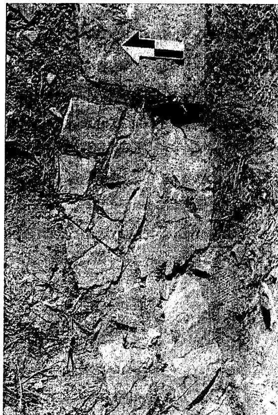
Figure 14: Feature 1, foundation wall between Rooms A and B showing tracked vehicle damage
