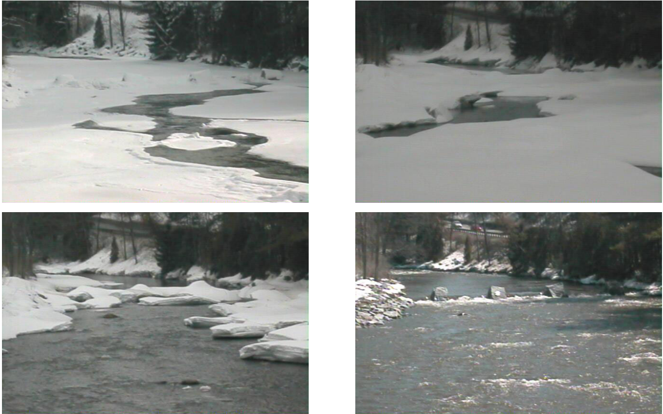
Figure 3. Images of the Hardwick Ice Control Structure showing different ice cover conditions.
