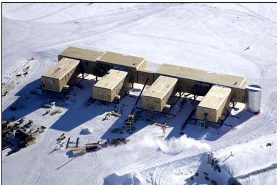
Figure 17. Downwind view of the Elevated Station showing the clutter associated with construction activities. This photo was taken on 24 January 2005. Note that, compared to Figure 7, the snow ramp has been removed and the superstructure of Wing's A4 and B4 are in place. The view is along the 0° meridian (true north).
