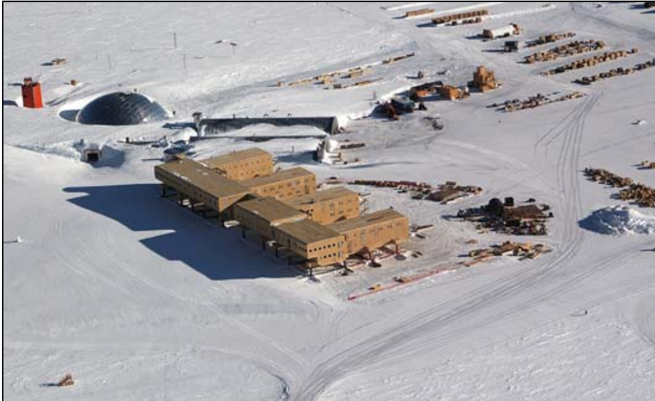
Figure 1. Elevated Station, the centerpiece of the Amundsen-Scott South Pole Station as it appeared on 29 January 2005. The exterior cladding had not yet been applied. The geodesic dome in the background was the centerpiece of the second Amundsen-Scott South Pole Station, constructed in 1975 and slated for disassembly over the next three years. This view is along the 150°E meridian.
