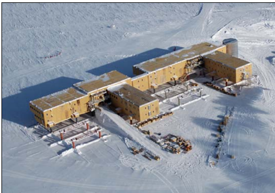
Figure 8. Snow ramp adjacent to the Wing B1 allowing direct delivery access to the loading dock on the back (downwind) of the B2 Wing. This photo was taken 7 November 2004, prior to completion of Wings A4 and B4 superstructure. The view is along the 45°E meridian.
