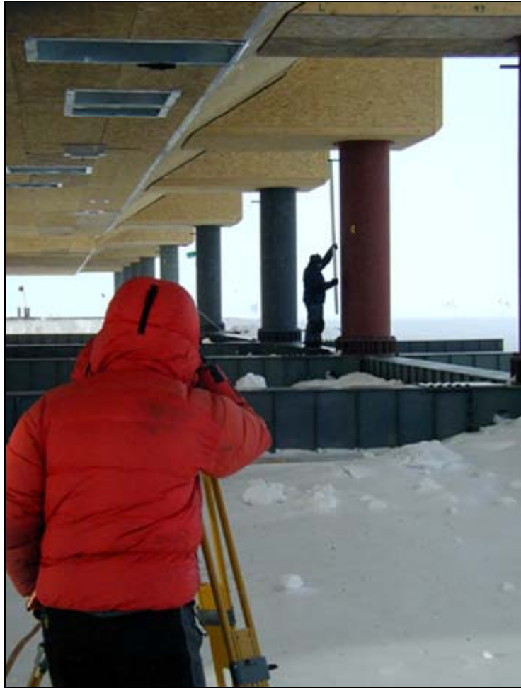
Figure 3. Workers collecting column elevations as part of a monthly survey during the austral summer field season. Note the welded tab protruding from the top of each column, from which the survey measures column elevations.
