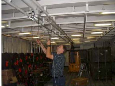
Figure 7. Ship Magazine on the USS Harry S. Truman: A member of the TM staff installed wiring for the RFEs.
