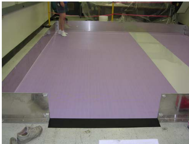
Figure 15. Decal as Seen During Installation
