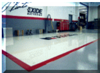
Figure 6. Typical Epoxy Floor (From Ref. [8])
