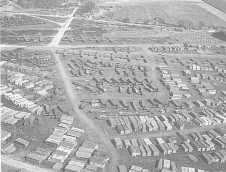
Glider assembly: CG-4As (Wacos) in wooden crates, foreground; fuselages out of the boxes, middle; assembled gliders at top. (Courtesy Smithsonian Institution)
