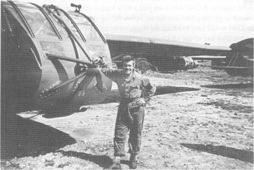
Hard-nose glider: Tazewell Sanderson (glider mechanic) displays the "Griswold Nose" modification to help Waco glider pilots deal with hedges and other obstacles when landing.
