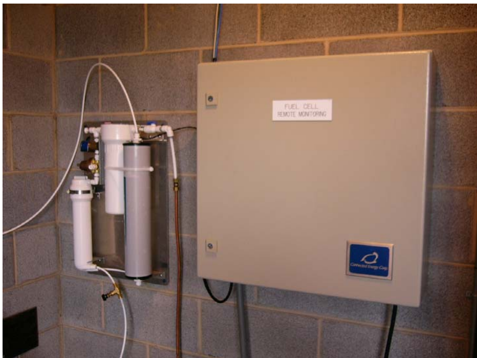
Figure A1. Water filtration system and communication and data acquisition box at Fort Gordon.
