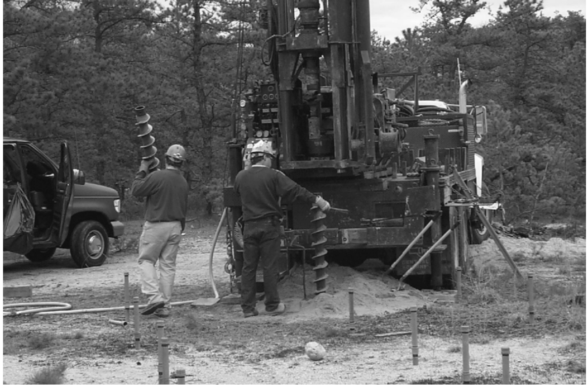
Figure 7. Rotary drilling rig (CME-75) with 6-in-OD hollow-stem augers used to install 2-in-diameter observation wells.
