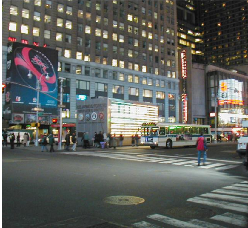
Figure TS.1—Times Square Station Exterior
