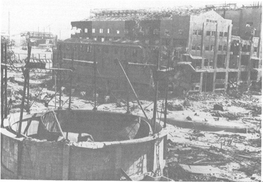
ALL THAT REMAINS OF THE POWER AND GENERATOR PLANT at the Imperial Fuel Industry Company at Ube, after the bombing attacks of July and August 1945.
