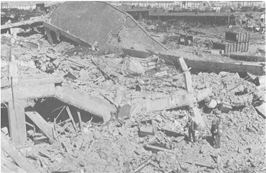
THREE AMERICAN OBSERVERS examine the twisted ruins of the Kugelfischer ball-bearing works at Schweinfurt, bombed repeatedly by Allied forces.
