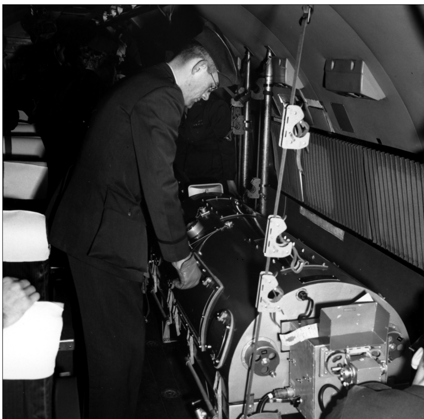
An iron lung is secured for flight on a C-130 cargo plane. (NARA photo.)
