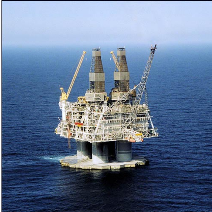
Figure 1. The Hibernia oilrig is located in the Jeanne d'Arc Basin, 315km east of St John's, Newfoundland, in water 80m deep.
