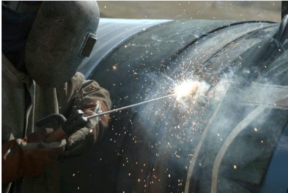
Figure 3. Finished pipelines in Iraq are constructed of schedule-40 black steel and assembled in 40-60 foot sections for above-ground use. [SPG Media Limited, 2005]
