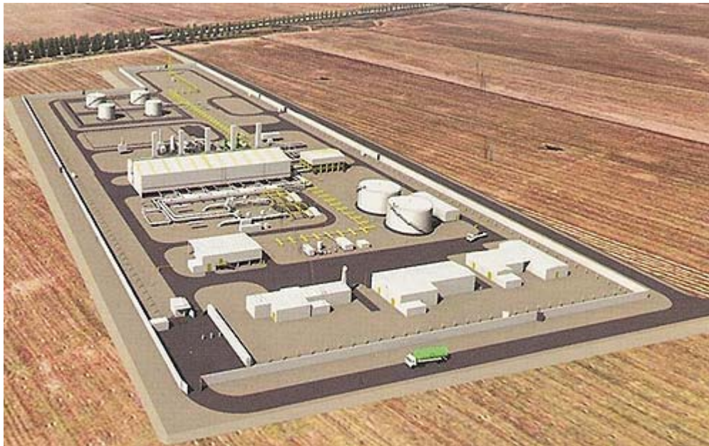
Figure 6. Artist's representation of a typical pump station with ancillary facilities. [SPG Media Limited, 2005]. Pump and booster stations similar to this are typically groupings of pumps operating in parallel. They are constructed approximately every 90 miles and their cost is a function of the expected flow capacity (gallons of oil per minute). This results in costs ranging from $0.25 to $9.8 million dollars per station in Iraq.
