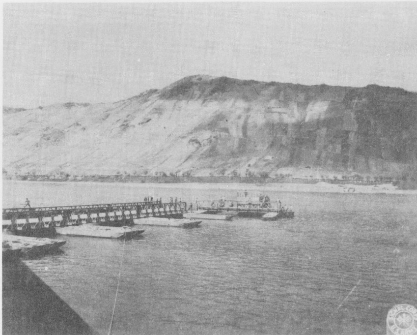
Photo No. 39 FLOATING BAILEY BRIDGE UNDER CONSTRUCTION AT LORCH.
