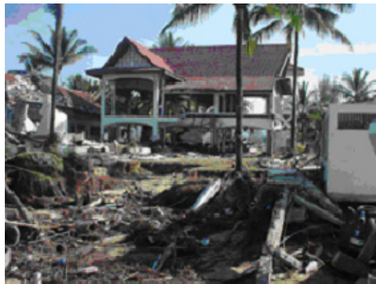
Figure 6. The hotel after the tsunami
