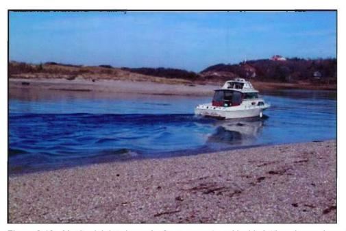
Figure 2-10. Mattituck Inlet channel, after turn eastward inside jetties. Large deposits of gravel and sand line both sides of channel, 21 November 2003
